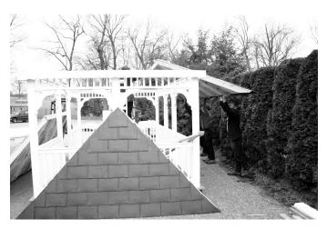
21. First raise a long side panel up onto the top plate. Slide this section up until the rafters in the roof drop into the top plate while resting against the inside of the fascia.
