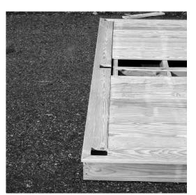
6. Now you will want to set the missing top decking boards into place, you will notice that they also have letters for proper placement. You will want to screw these decking boards into place with 2 ½" screws. (If you have composite decking you will use the screws that are the same color as the deck)
