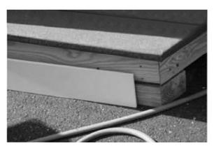
27. Gather all of the bottom fascia trim boards and place them along the bottom of the decking. Find the center of each deck side then, find the center of the corresponding floor trim board.
