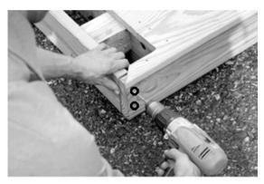
5. Next you will take the two decking ends that were removed earlier and you will want to screw them into place with 3 ½" screws. Screw the deck ends to the outside of the deck frame. After you have connected the exterior of the floor frame together you can now go back and tighten the bolts you set into place in the previous step.
