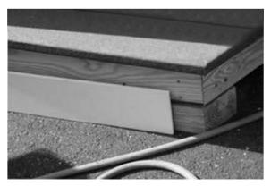
41. Gather all of the bottom fascia trim boards and place them along the bottom of the decking. Find the center of each deck side then, find the center of the corresponding floor trim board.
