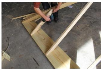
16. The jack rafters are only be able to fit into one location. Take each one and the hold it in place with the tops against the side of the center rafters, and the bottoms against the top plate. Once fit snugly into place, take a 2 ½" screw and connect the top of the jack rafters to the center rafters. Connect all of the jack rafters at the top first.
