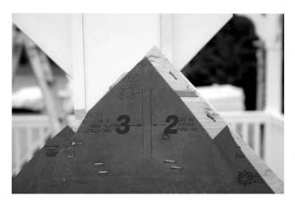
20. You will notice that all of the roofing sections are labeled and have two numbers on them. You will want to find the sections with the same numbers and match them together. Also you will notice that some of the roofing sections come to a point at the top and the others are flat. The sections with the flat ends are the longer sides of the front and back. They go together first.
