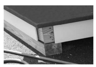
28. Line up the center marks and fasten the trim board to the outside trim board with six 2 ½" white head screws. Use two screws on each end and two in the middle. Do this all the way around the gazebo. For larger gazebos, fasten with two screws every 3 feet.
