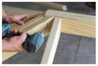
14. Then take the tops of the corner rafter and set them against the ridge board as shown. Once in place, screw them into the top plate with 2 ½" screws two from each rafter into the top plate. Do this until all the corner rafters are installed.
