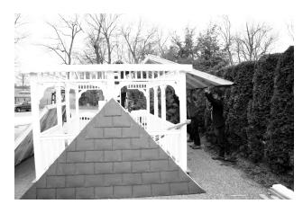
33. First raise a long side panel up onto the top plate. Slide this section up until the rafters in the roof drop into the top plate while resting against the inside of the fascia.
