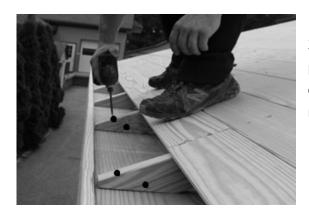
39. Use 2 ½" screws to attach the rafters to the top plate. You will want to screw one screw into the top of each rafter and then also one into the side of each rafter.
