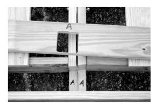
3. You will notice that there are letters on each joist that will join to another numbered or lettered section. Arrange each section with these numbers/letters as shown. Also the deck boards will have corresponding letters.
