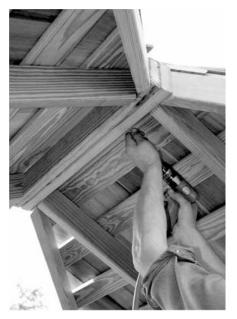
36. Once you have both sections set into place, you will need to raise both panels so they mate at the ridge. Make sure that you have a helper tending to the props so that they do not get dislodged during this process. With the roof panels aligned and flush with each other, you will want to secure them together with 2 ½" screws. At this time please do not attach the rafter to the top plate.
