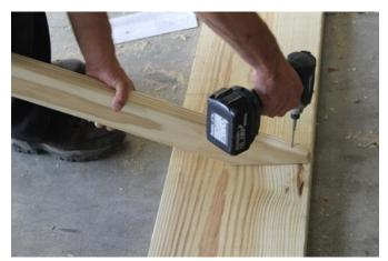
18. Now that the jack rafters are set in place with the correct spacing, screw them into the top plate with 3 ½" screws, one in the top of each rafter and one through the side. Follow this process until all of the jack rafters are installed.
