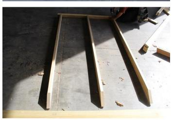
3. Next, find the center ridge rafters, these boards will be the same length and will have a matching angled cut on both ends like the picture shown. Make sure that the boards are laid out on the ground as shown.
