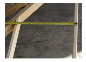
17. When they are all connected at the top, take a measurement from one jack rafter to the next at the top. This measurement will allow you to know how far apart the rafters should be spaced at the bottom.
