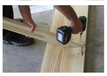
11. Next, attach the bottom of this rafter to the top plate as done with the other rafters, using 3 ½" screws one through the top and one through the side. Follow this process for the other side as well.
