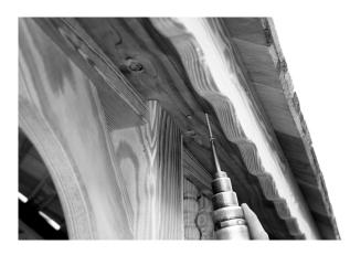
26. To fully secure the rafters to the top plate you will need to drive a 3 ½" white headed screw from the bottom of the top plate up into the rafters. You will want to insert the screws 1" from the outside edge of the top plate. Do this around the entire Gazebo at every rafter. The roof is now complete and is ready to have the ridge capping installed.
