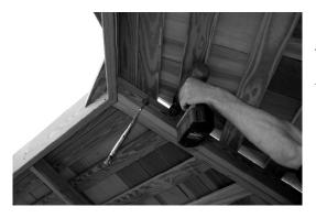
Tip: You can use several aides in aligning the rafters. A clamp is very handy in keeping the rafters aligned until they are secured to each other.
