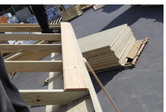
19. After, all the jack rafters are fully installed it is time to install the T&G roof decking. The structure will come with a bundle of T&G decking boards. Start at the bottom of the roof and work your way up to the top with them. Cut these boards to size before they are installed.
