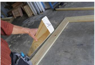
9. After, fully securing all of the center rafters to the top plate on both sides of the roof, install the singular center rafter for the other side. This normally will be the short side if applicable. The rafters will be labeled with a letter on the cut along with the matching letter on the end of the ridge boards. As shown in the picture to the left.
