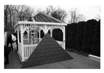
35. After you have the first section in place you can use a prop board to hold it into place while you get the second long side roofing section set into place. If you use a prop make sure that you place it toward the inside of the roof panel, so you do not have the chance of it see-sawing.
