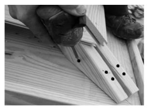
38. Once you have attached all the roof panels together, the next step is to attach the rafters to the top plate. This is why you removed those bottom boards earlier!
