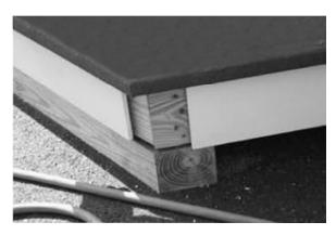
42. Line up the center marks and fasten the trim board to the outside trim board with six 2 ½" white head screws. Use two screws on each end and two in the middle. Do this all the way around the gazebo. For larger gazebos, fasten with two screws every 3 feet.
