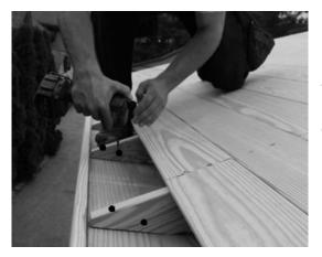
40. Once all of the rafters are attached to the top plate, you can now re-attach the roofing boards that you previously removed. And now you are ready to install shingles on the roof.
