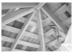
25. Next raise an adjoining panel into position, a prop is handy in aligning the end panel with the main panel. Keeping the end panel/rafter flush with the adjacent panel/rafter, secure them every 24" using 2 ½" screws. Continue this until all roofing sections are installed and secured.
