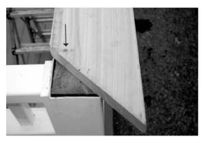
14. Screw in a single screw on one end of the top plate to hold it in place while you are positioning it. Now once it is in place on the other end put a screw in that side as well to keep it in place. Screw only the first board down at this time.
