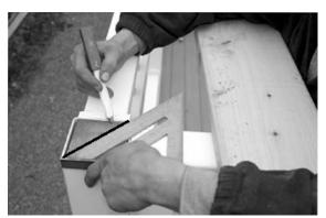
13. Next you want to install the top plate boards. Take a straight edge and drawing a line dividing the top of the post diagonally. Position the first top plate board along that same line and make sure that you have a ¼" overhang toward the inside of the Gazebo at each post.
