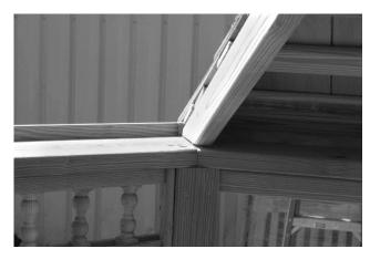
34. Align the rafters with the edge of the top plate, resting against the fascia.
