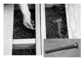
4. There will be holes in the deck joists where they connect together with  $\frac{1}{2}$ " x 4" bolts. For the moment you will just want to put the bolts in place and finger tighten them. You will finish tightening them after the next few steps.
