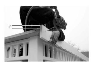
16. Now you can install the outside fascia. You will need to make sure that the fascia sets up 1" above the top plate. Once the fascia is in position you will want to screw it into the top plate with 2 ½" screws every 24". The screws should be 4" in from each end and 1 ½" to 1 ¾" from the top edge. Also the fascia may be a little long and will need to be cut to size.
