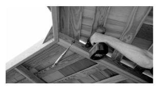
Tip: You can use several aides in aligning the rafters. A clamp is very handy in keeping the rafters aligned until they are secured to each other.
