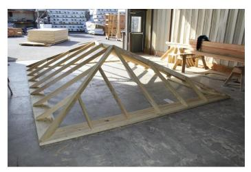
1. After you have installed the top plate and fascia boards, you are ready to start the installation of the stick built roof. To the left is an image of a 12' x 14' stick built Hip roof frame. This was built on the floor without the fascia.
