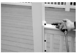
11. Now you can install the bottom railing sections. You will need to set these sections into place and center them on the posts. Make sure that the bottom of the rail sections are touching the decking below. Once the section is in place you can screw it into the post with 4 - 3 ½" white head screws. You will continue this until all bottom rails are installed.
