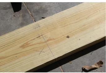
5. When this is done for both sides of the center sections, look at the top plate board and see another set of X's with lines beside them. This will be your guide as to where the other ends of the rafters that were just connected to the ridge board, will then be connected to the top plate.
