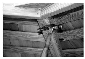
Tip: Also to pull a panel into position for alignment you can drive a screw into the higher panel/rafter and using the claw on a hammer pull it down into position.
