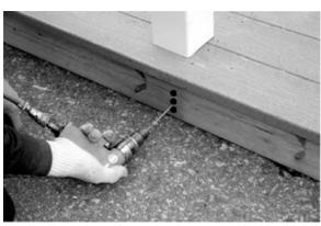
17. Now that both the top and bottom rails and top plate with fascia are installed you will want to go around the bottom of each post and secure the frame of the deck (rim board) to the posts. You will do this by screwing three 3 ½" screws into each outside facing post. This is very important because it will provide a lot of the stability for the Gazebo.
