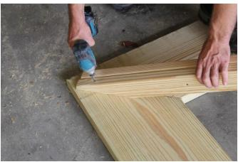
13. Next, set the bottom of these two boards centered on the top plate and up against the fascia. Once in place, screw these rafters into the top plate with 3 ½" screws, one in the top of each rafter and one through the side. Follow this process for all four corners until all the bottoms of the corner rafters are attached.
