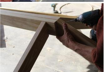
10. Now, take this rafter and place it on the center of the two ridge board ends, making sure that it is flush with the top. Then connect the rafter to the ridge boards with a 2 ½" screw from the top and one from each side.
