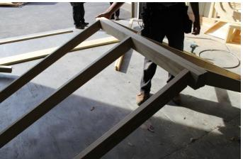
6. Next, take the ridge board and center rafter sections and rest the ridge boards of the two sections together. Once they are resting against each other, make them flush on the ends and also on their tops. (please use the picture at left as a reference)
