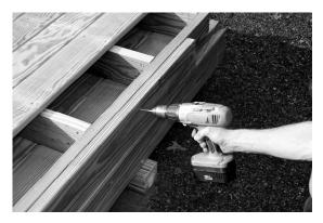
1. The first thing you will need to assemble is the floor of the structure. The floor is shipped to you in sections. Typically there are 2 floor sections but the floor may come in 4 floor sections for larger Gazebo's. You will need to first remove the boards attached to the end of the deck sections. (These will be used in Step #5)
