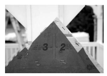
32. You will notice that all of the roofing sections are labeled and have two numbers on them. You will want to find the sections with the same numbers and match them together. Also you will notice that some of the roofing sections come to a point at the top and the others are flat. The sections with the flat ends are the longer sides of the front and back. They go together first.
