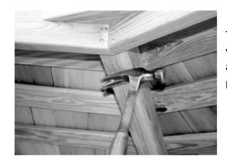
Tip: Also to pull a panel into position for alignment, you can drive a screw into the higher panel/rafter and using the claw on a hammer pull it down into position.
