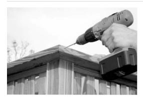
15. Position the adjoining top plate for installation and screw it from the corner to the other top plate. Follow these steps until all the top plates are in place. Make sure all corners fit tight and are spaced evenly over posts. \*You may need to un-screw the first board to get the tight fit. Then you will want to fully secure the top plates from the top by driving a screw every 16" the entire length of the top plates with 2 ½"
