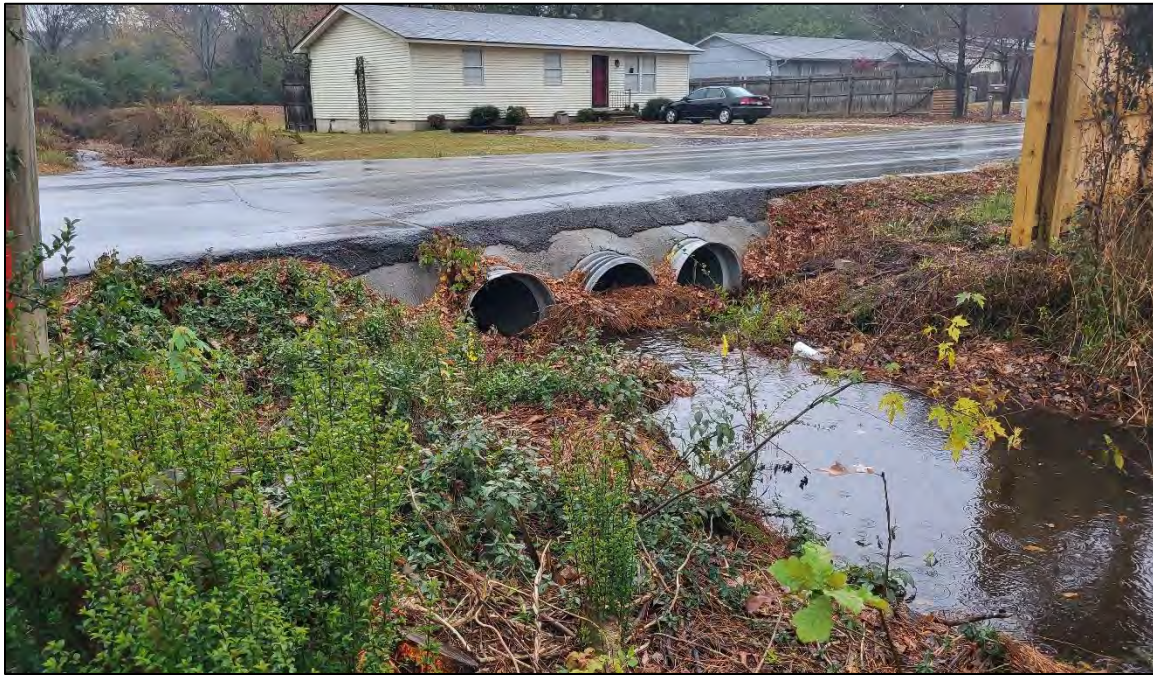
Figure 4. Upstream face of culverts at Boone Road
