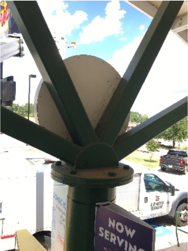
EXISTING SIGN- TO BE REMOVED/BACK VIEW OF BRACING
