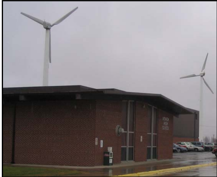
* Turbine 1 on left and Turbine 2 on right.
