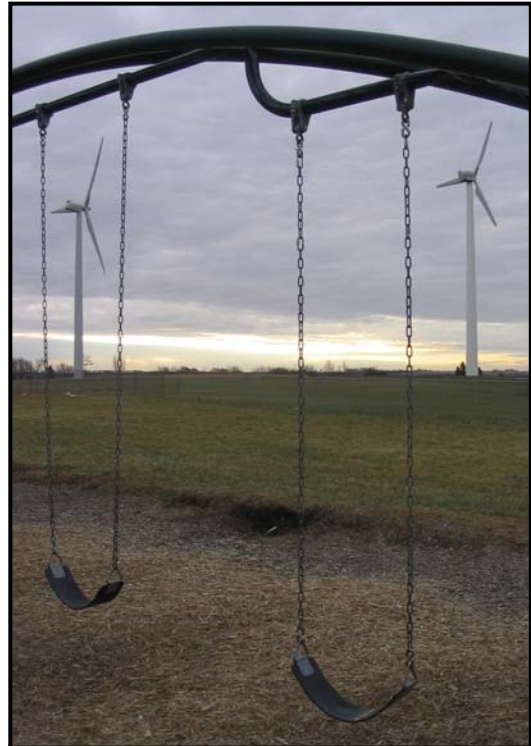
* Turbine 1 on right and Turbine 2 on left.
