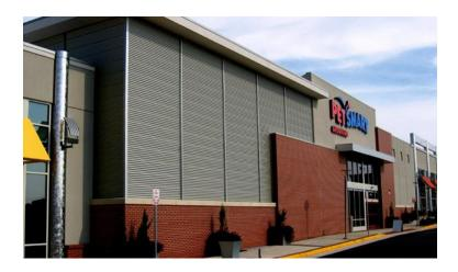
L. Metal Siding with a sine wave pattern (May not exceed 30% of total area of any one façade)
