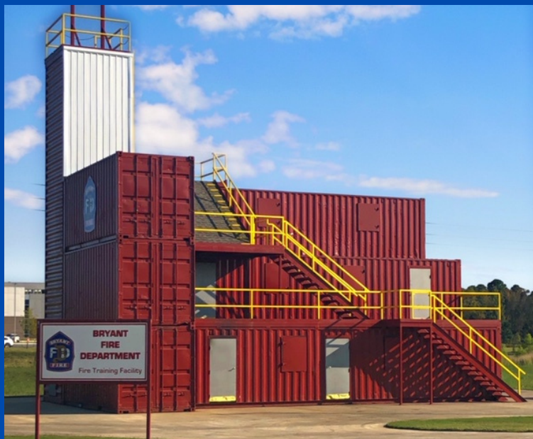
Bryant Fire Department Fire Training Facility
