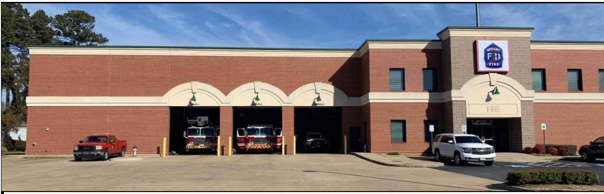
Fire Station 1 located at 312 Roya Lane
