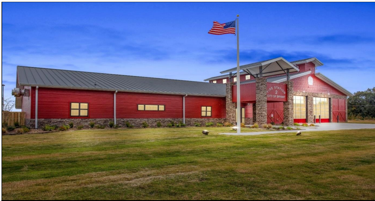
Fire Station 2 located at 1601 South Reynolds Road
