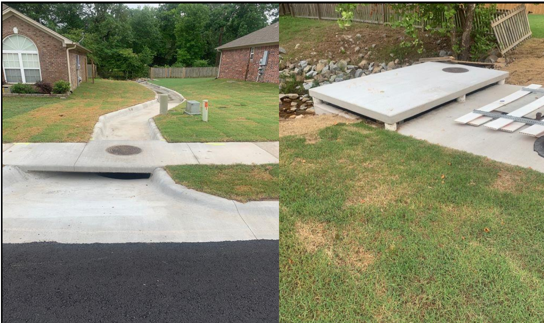
Drainage improvements completed in 2019
