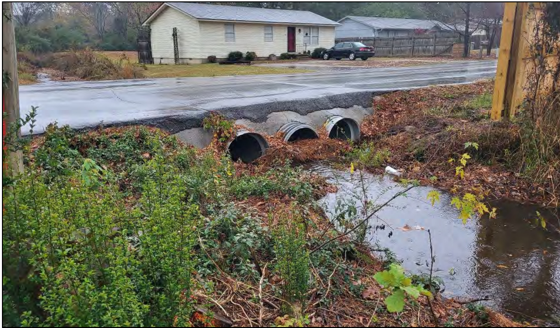
Figure 4. Upstream face of culverts at Boone Road
