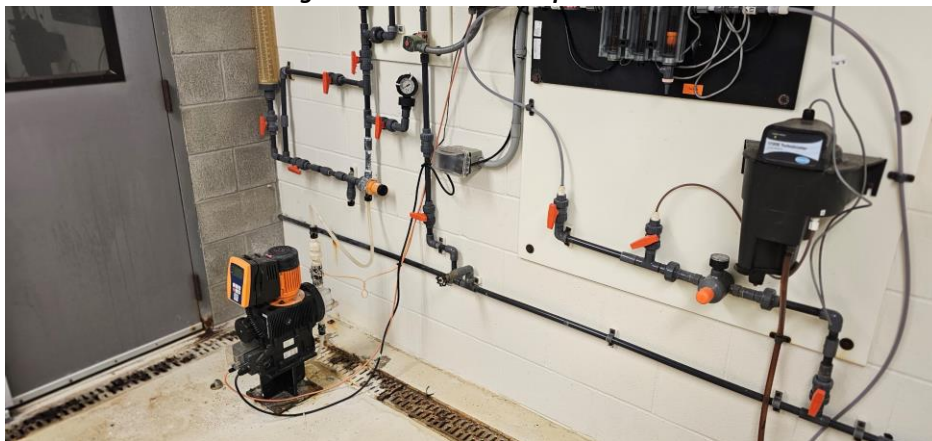
Figure III-4: Chlorination Unit with Corrossion Evident
