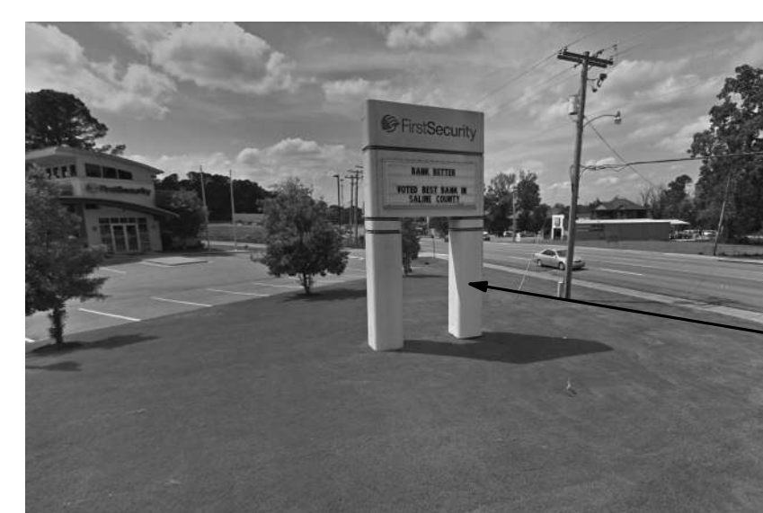
EXISTING PYLON SIGN TO BE REMOVED IN ITS ENTIRETY. EXISTING ELECTRICAL UTILITIES TO BE CAPPED AND CLEARLY MARKED FOR FUTURE USE
